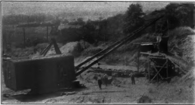
Excavating Asphalt Filler
